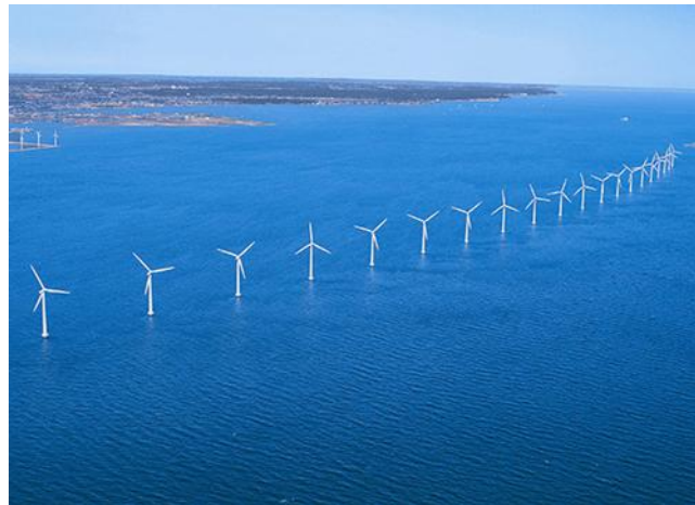
Fig. 3. Offshore wind. Offshore wind is 50% stronger and steadier than land-based wind, and requires shorter transmission distances. Superconducting wire enables high output, low weight wind turbines, reducing the cost of offshore wind to competitive levels. Source: Earthyreport.com
